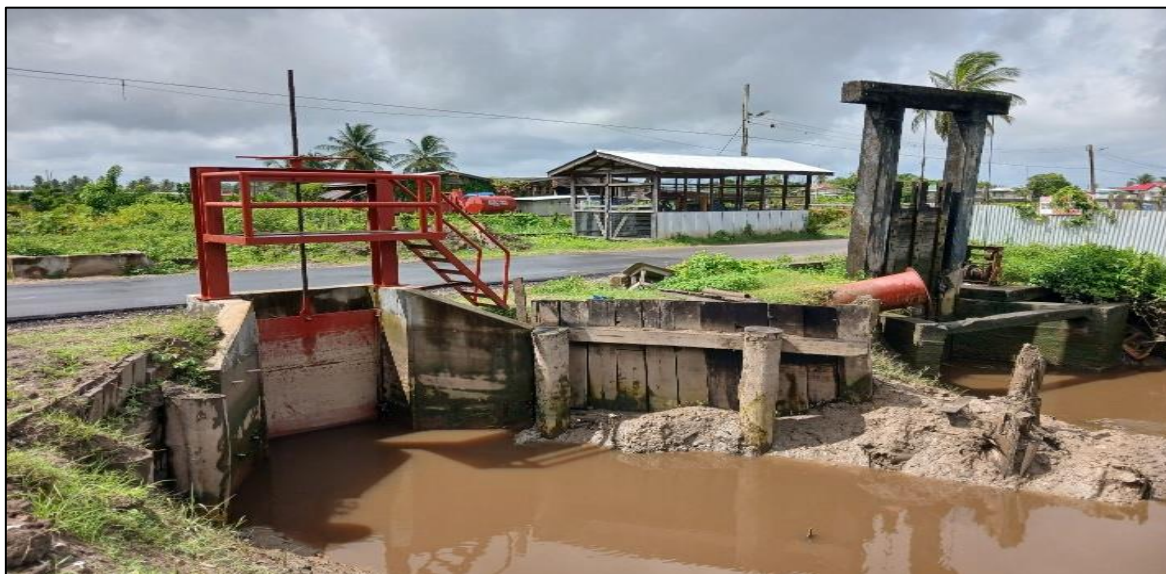
Fig 2 Lot 31 Old (Right) and Newly Constructed (Left) Lot 31 Sluices and Pump Station in Background.
