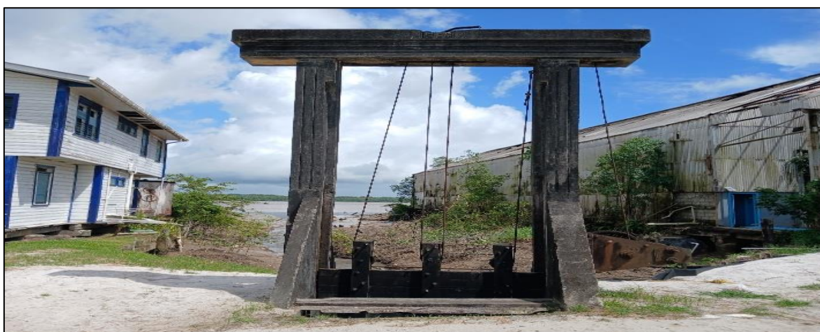
Fig 3 Lot 51 Sluice Discharging by Gravity During Low Tide.
