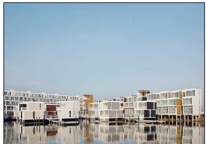
Fig 4 IJburg Floating Houses (Source: https://www.archdaily.com/120238/floating-houses-in-ijburg-architectenbureau-marlies-rohmer )
