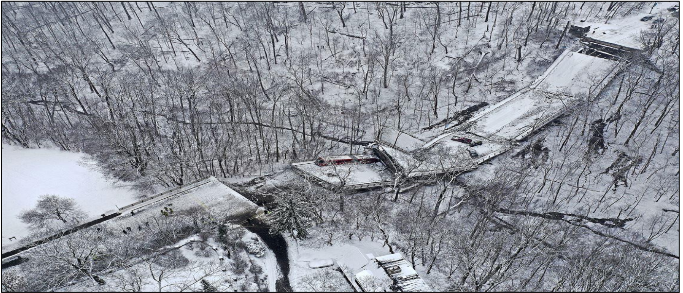
Fig 4 The Fern Hollow Bridge Collapse
