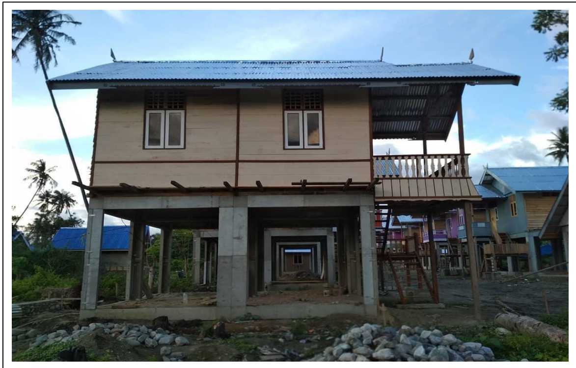
Fig 5 RISHA Huntap Panel for the West Mamboro Independent Relocation Area (ARKOM Documentation, 2024)
