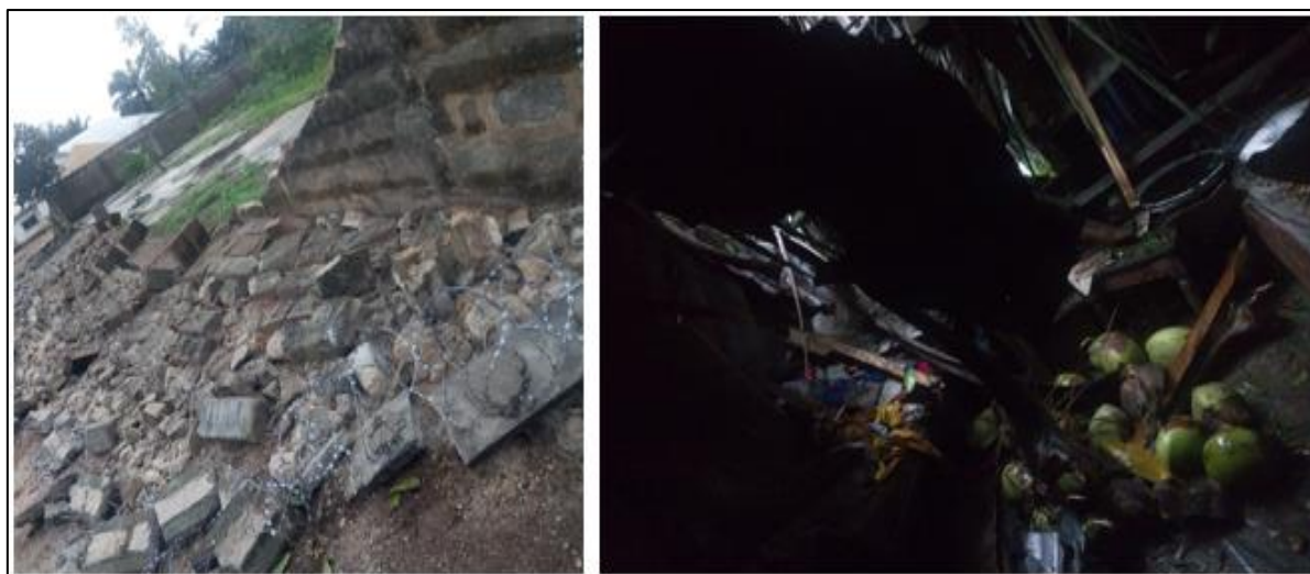
Fig 4 Flood Damage Observed in Residential Compounds Following the April 2021 Rainstorm.
