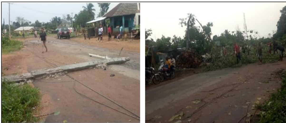
Fig 7 Damaged Electricity Infrastructure Along Major Routes, Including the Umuogide–Federal College of Land Resources Technology (FECOLART) Road.
