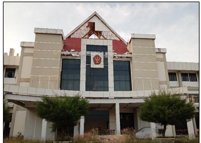
Fig 2 Existing Building of Tadulako University Hospital
