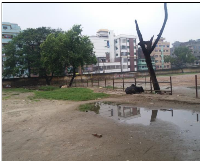
Fig 8 Lack of Proper Drainage System Causing Accumulation of Rainwater. Source: Authors' Field Survey.
