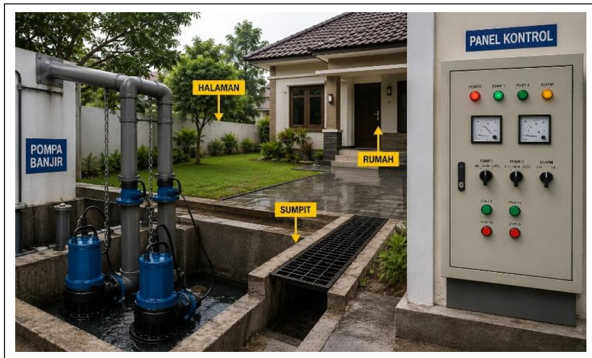
Fig 1 Ilustration of Flood Pump.
