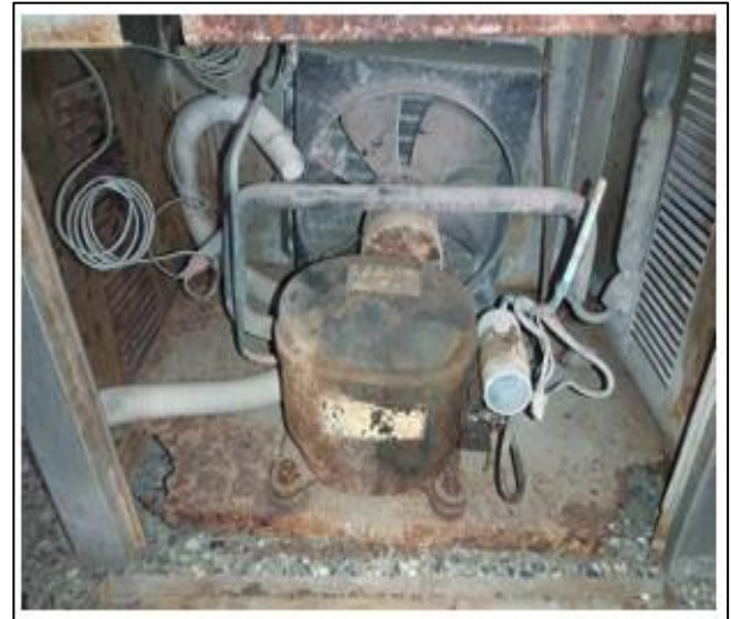
Fig 1 Internal View of Water Cooler before Restoration
