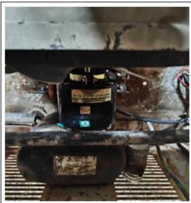
Fig 5 Installed New Fan Motor
