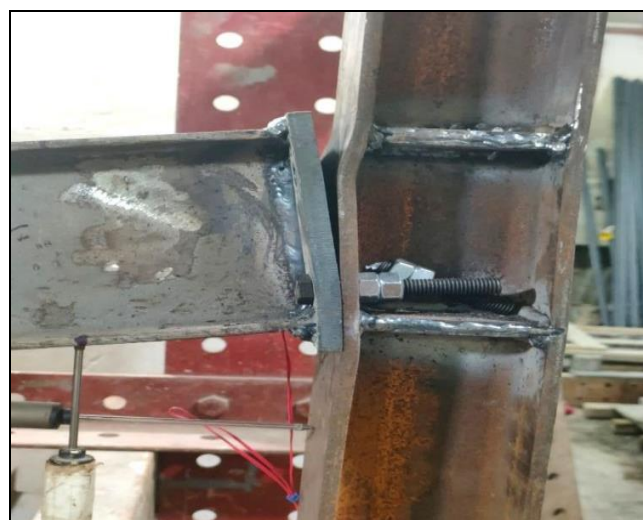
Fig 10 Deformation of Column Flange and End-Plate, and Bolts Failure in Specimen 2 at a Loading Distance of 45 cm
