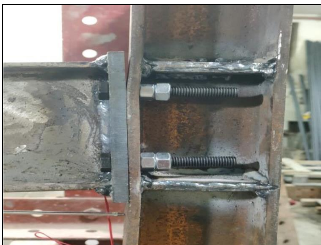
Fig 9 Column Flange Deformation of Specimen 2 at a Loading Distance of 25 cm
