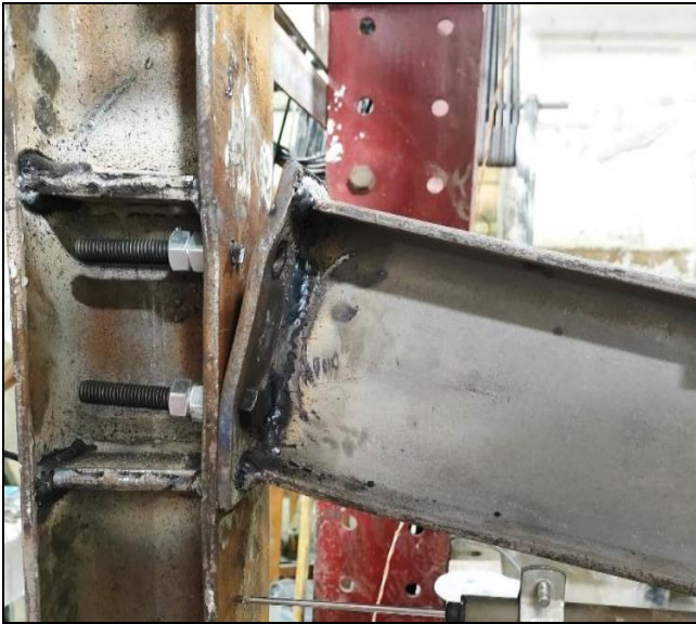
Fig 12 Deformation of Column Flange with End-Plate and Bolts Failure in Specimen 3 at 25 cm Loading Distance
