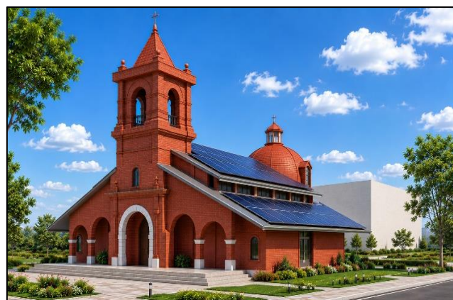
Fig 22 Energy System with Rooftop Photovoltaic Panels.
