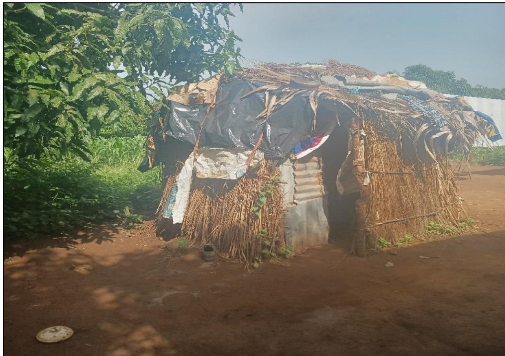
Fig 6 Example of Local Construction Observed on the Site.
