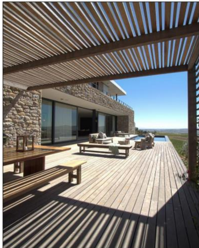
Fig 4 Brise-Soleil Terrace. Source: Archzine [23].
