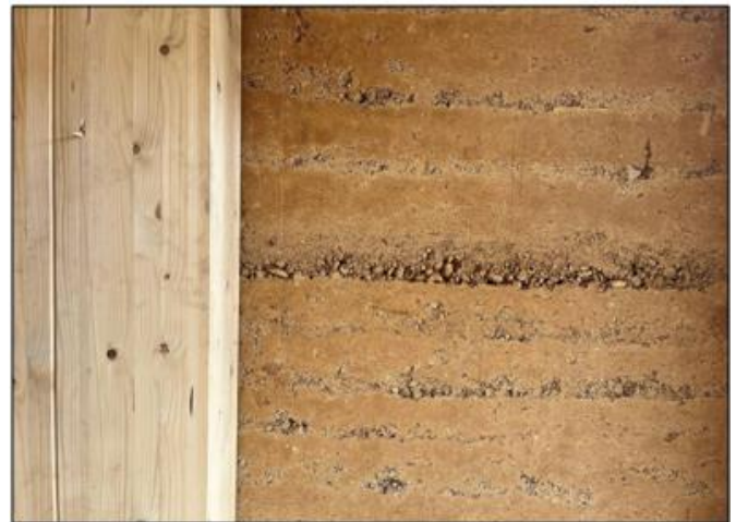
Fig 12 Raw Earth Wall and Timber Surface. Source: Mil-Lieux [46].
