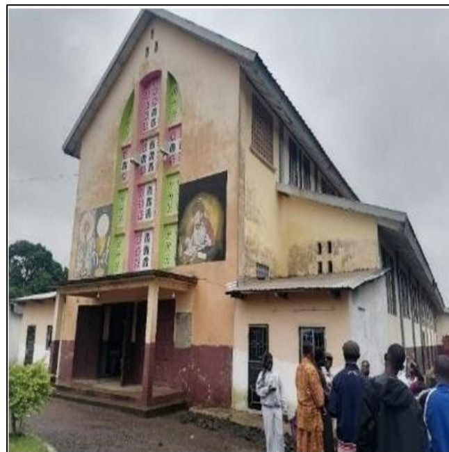
Fig 7 Main Façade of Saint Luc Church in Njombé-Penja During Renovation Works.
