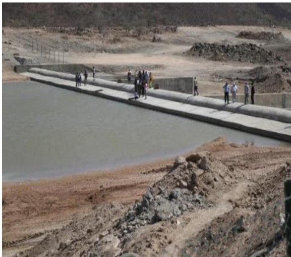
Figure 4.1 Humba-Wayne Rain Water Irrigation Dam (Source: Field Survey 2019)
