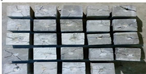
Figure – 4. Crack Pattern
