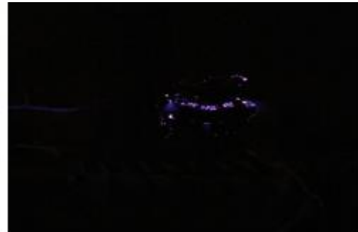
Figure 6: Corona formation on 11KV porcelain insulator at 50KV under wet condition
