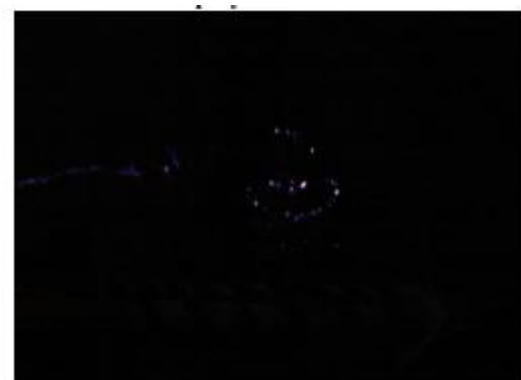
Figure 8: Corona formation on 11KV polymeric insulator at 50KV under wet condition
