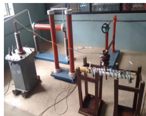
Figure 2: Setup for transformer to porcelain insulator
