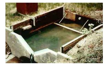
The picture above shows a V-notch weir. The edge the water cascades over is called the crest and the overflowing water sheet is called the nappy. Today weirs are still used to determine flows from open water sources such as streams. A typical 90° V-notch will be beveled at 45° so the edge is less than 0.08" thick and the angle of the notch will be precisely 90°. Water flow over the weir is calculated by the equation:
