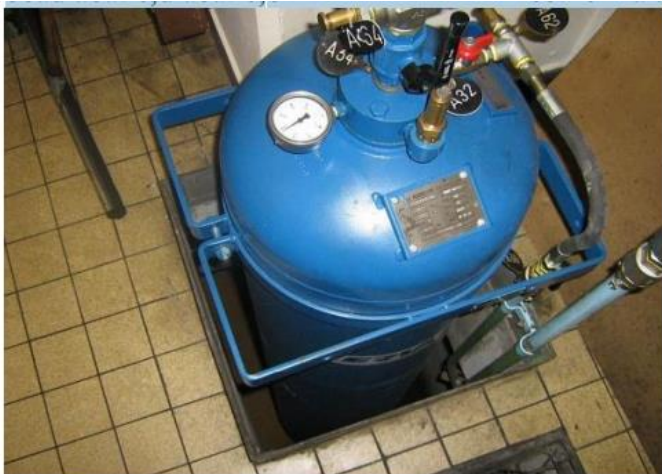
Fig: 2:- Storage Tank[1]
