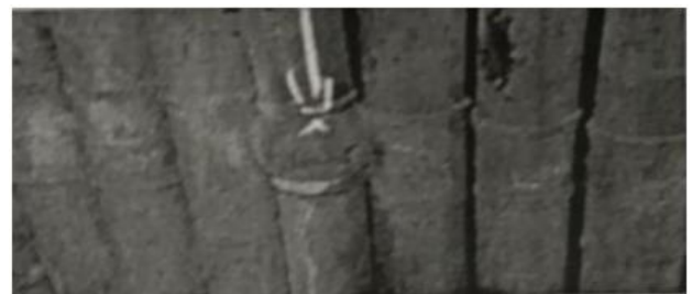
Fig 3:- Dissimilar Welded Joints
