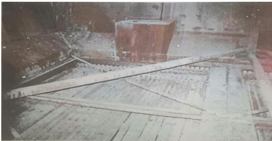
Fig 2:- Air pre-heater tubes corrosion
