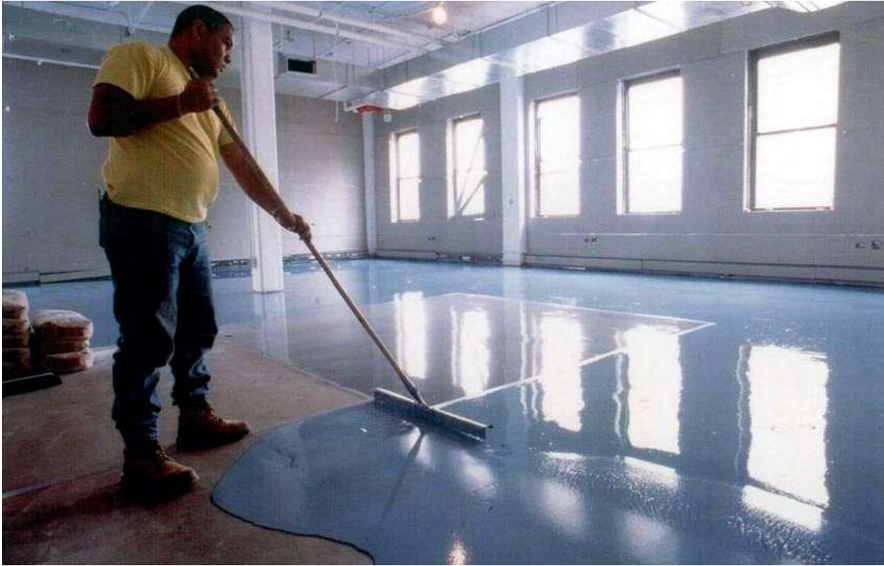
Fig 6:- Seamless Epoxy Floor Resurface Covers Damaged Floors
