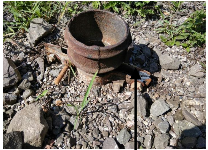
Fig.2:- Earthing system at substation
