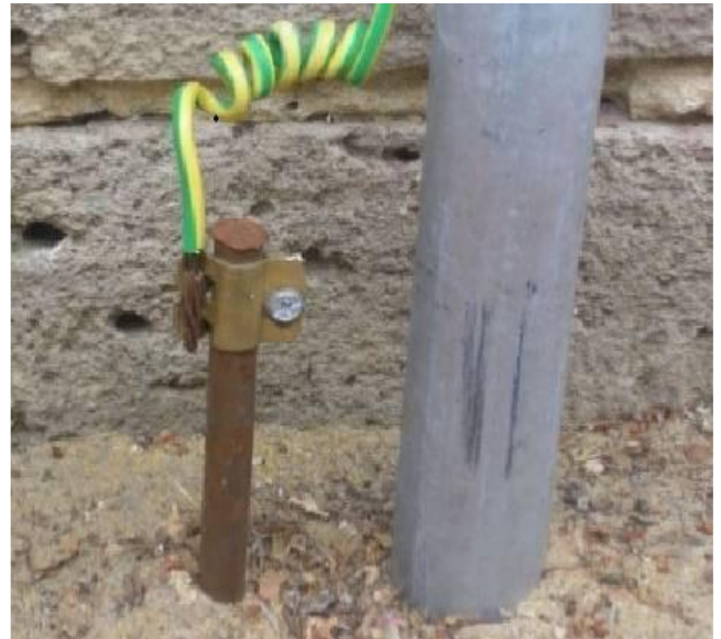
Fig.1:- Earthing system
