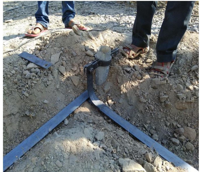
Fig 5:- Design Earthing system at 33/11 KV Pandare substation
