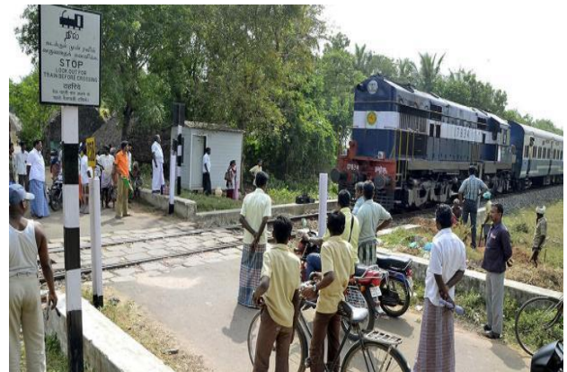
Fig 3:- Unmanned Railway Crossing
