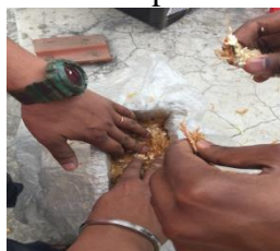
Figure 3.9 filling in the Brick mould
