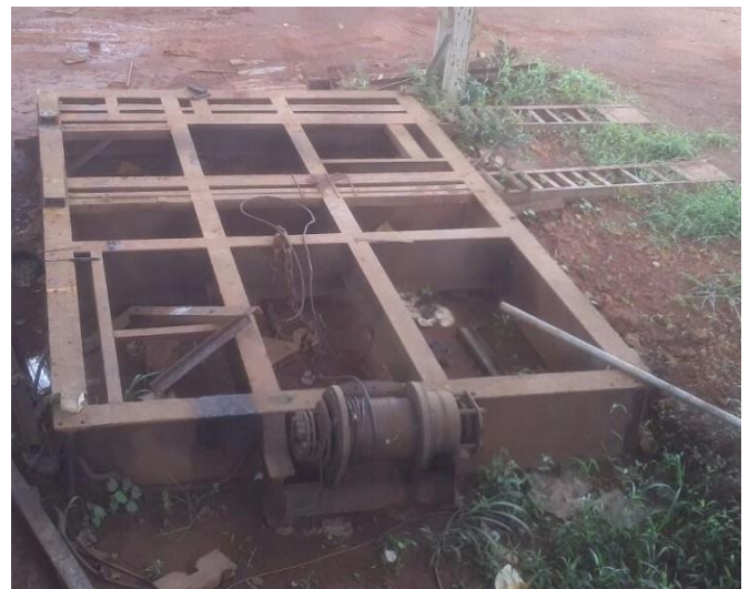
Fig 5:- EOT crane on platform one side
