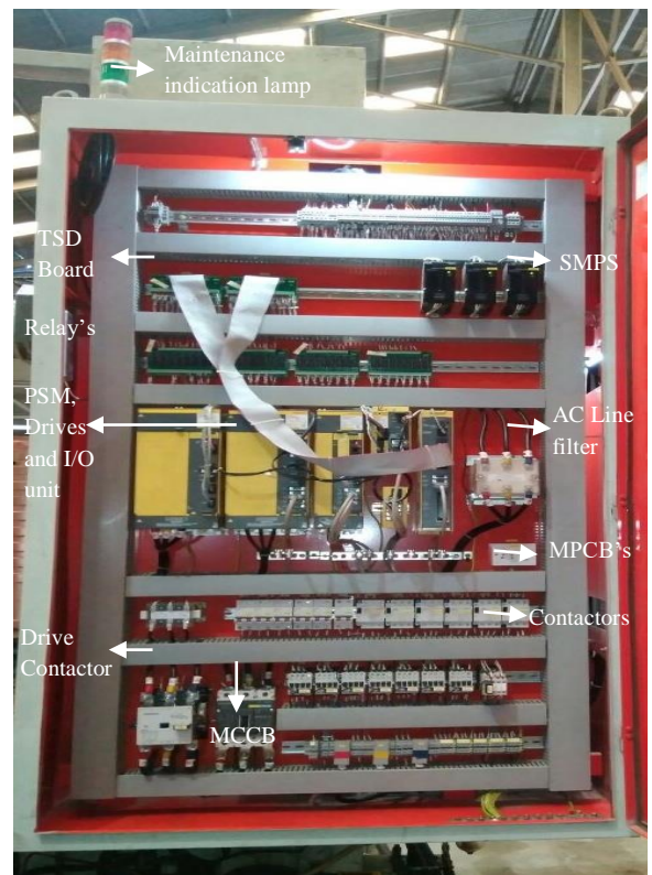
Fig 8:- Control Panel components Assembly
