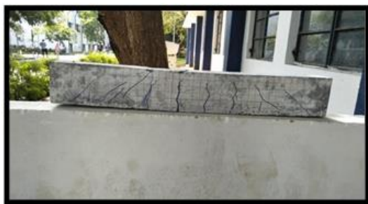
Fig 8:- Shear crack at specimen C1
