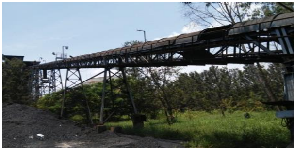
Fig 4:- Crushed Coal to furnace
