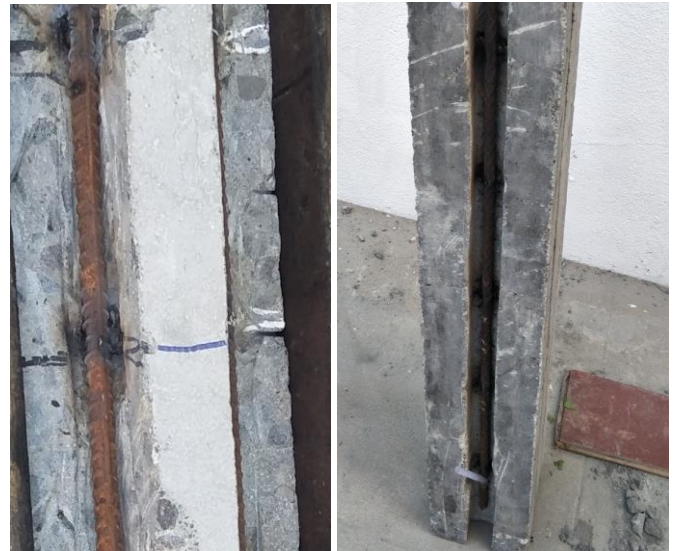
Fig 2:- Column cover removed and steel rods welded for retrofitting
