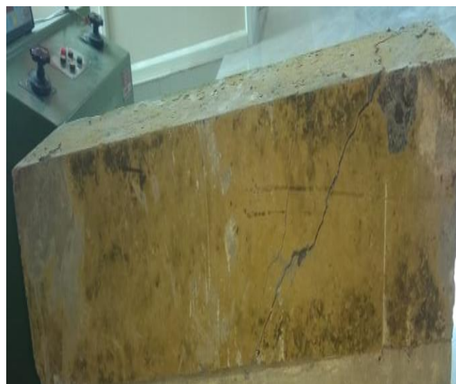
Fig 5:- Cracks development in Torsion (BFRP)
