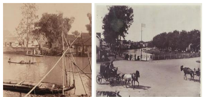
Fig 2:- Kalimas river and Peneleh bridge in 1880s(Source: http://hdl.handle.net/1887.1/item:788089 and http://hdl.handle.net/1887.1/item:788073 )
