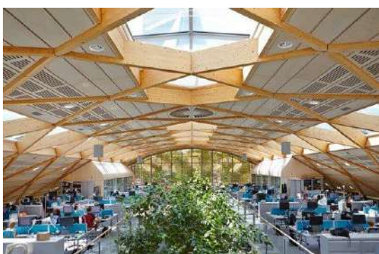
Fig 6:- Timber Diagrid structure
