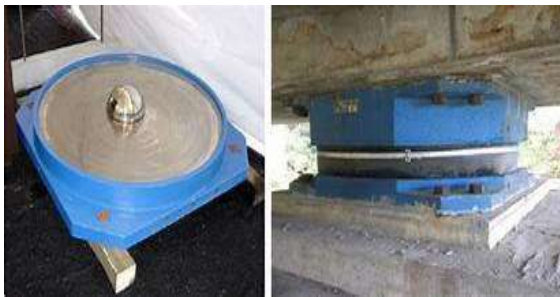
Fig 13:- Friction pendulum applied on a structure
