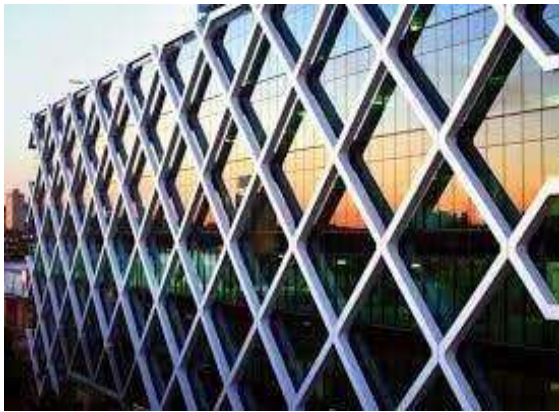
Fig 4:- Steel Diagrid structure
