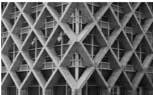
Fig 5:- Concrete Diagrid structure
