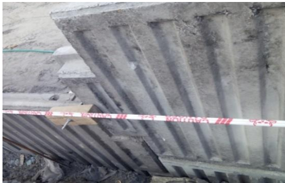
Fig 3:- Panel placement for initial course
