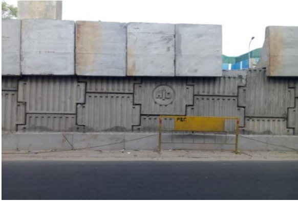
Fig 2:- Precast RE wall panels
