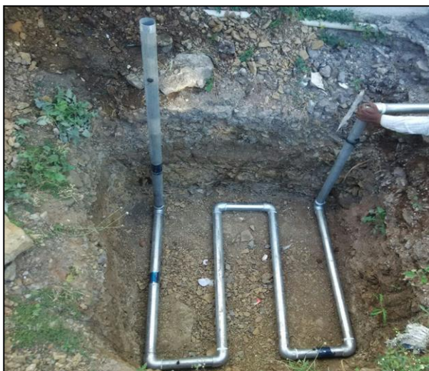
Fig 2:- Installation Pipe structure on Project Site
