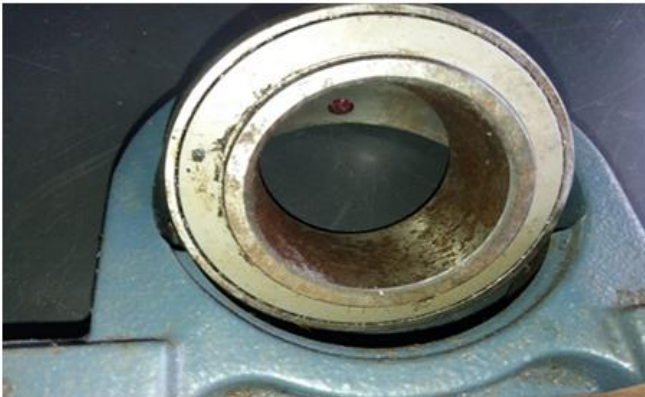
Fig 9:- Damage to Bering
