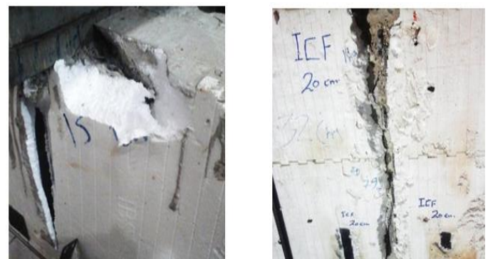
Destruction of the upper part under Loading
