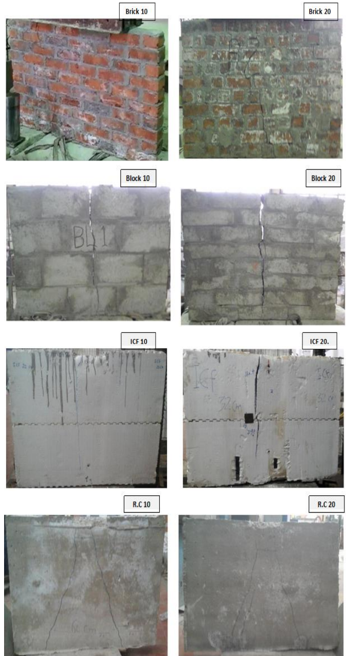
Fig 4:- Cracking Pattern and failure mode of the test specimens
