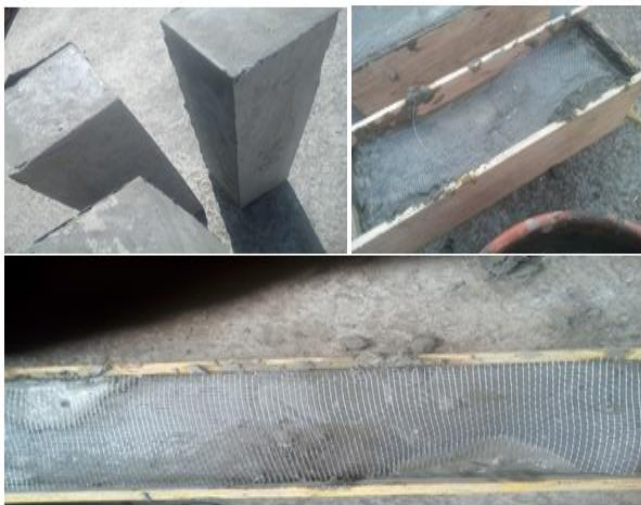
Fig 7:- Retrofitting And Reinforced Detailing Of The Beam.
