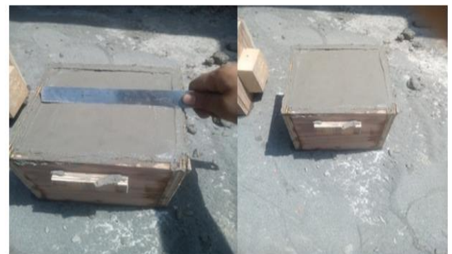
Fig 3:- Cubes Casting Process.
