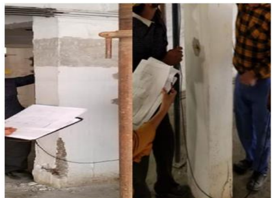
Fig 2:- Crushed Columns
