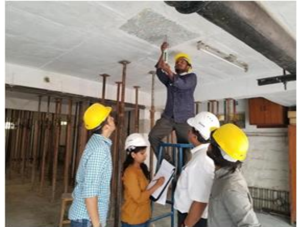
FIG 6: Rebound hammer test on Slab.
