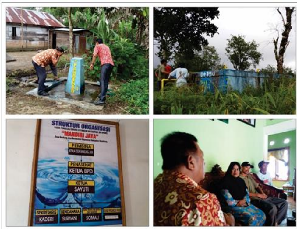
Fig 3:- Review of the organization and interviews with the management of BP-SPAMS Mandiri Jaya and review of the conditions of the Pamsimas infrastructure that are still well maintained.
